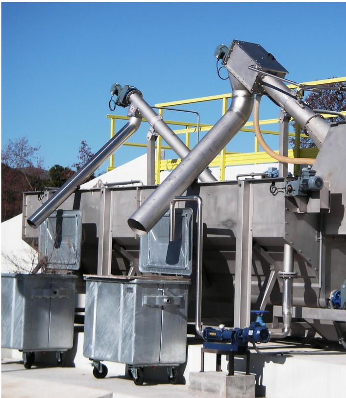
The Noggerath® Complete Headworks Unit (TOP) replace conventional headworks structures in wastewater treatment plants.
