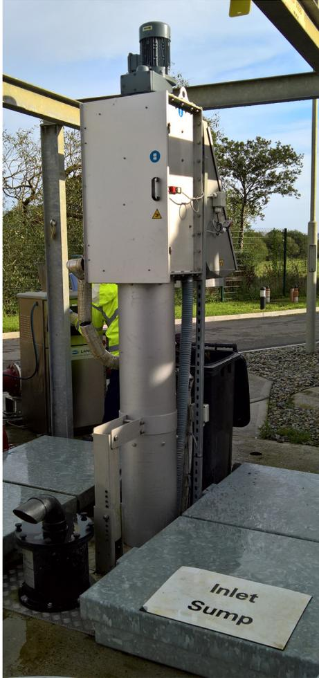
The Noggerath® Spiral Sieve Screen (NSI) is designed to be installed in municipal and industrial wastewater treatment plants. NSI screens provide the ability for small facilities to screen, wash, dewater and compact solids out of a waste water stream — whether it be municipal or industrial waste, improving the performance and reliability of downstream treatment processes.
