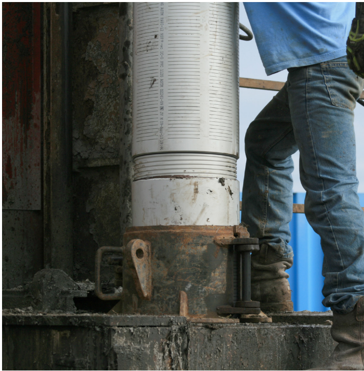
Shur-Grip flush thread allows for a quick assembly
