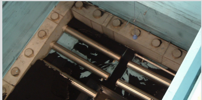
04 Off-set effluent collection/backwash water header 05 Center eductor 06 Sub-fluidized exhausted GAC media automatically educted from the basin
