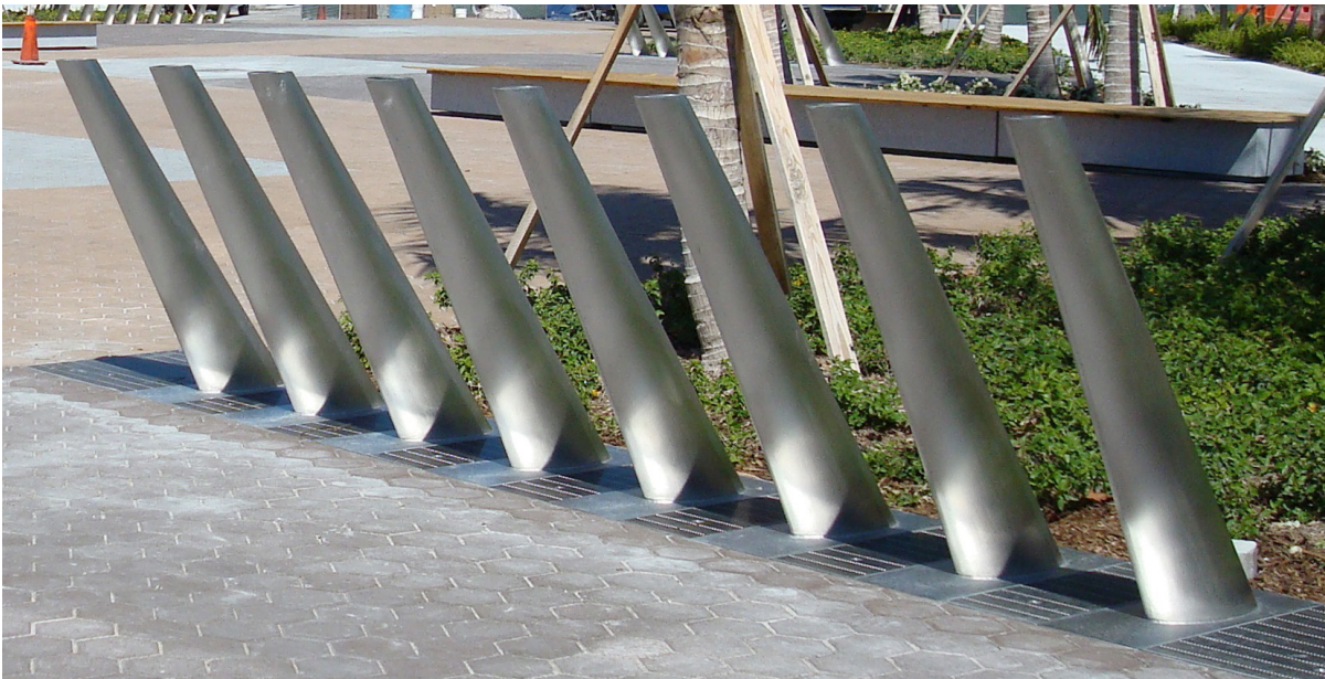
The 32 conical ellipse-shaped water jet shrouds are 48 in. tall and are made of 316L stainless steel. The shrouds are fitted with bulkheads that allow for an even stream of water to jet out. When the water comes out of the system, it arches over the pathways, creating an ever-changing experience for pedestrians as they walk through the park.
